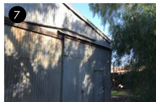
7 Back of Foundry
