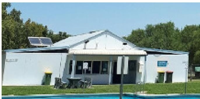
The amenities are constructed of brick with the kiosk in the middle and the amenities each side. They are in an average condition and will require a major upgrade to be DDA compliant. The kiosk requires a full internal refit.
