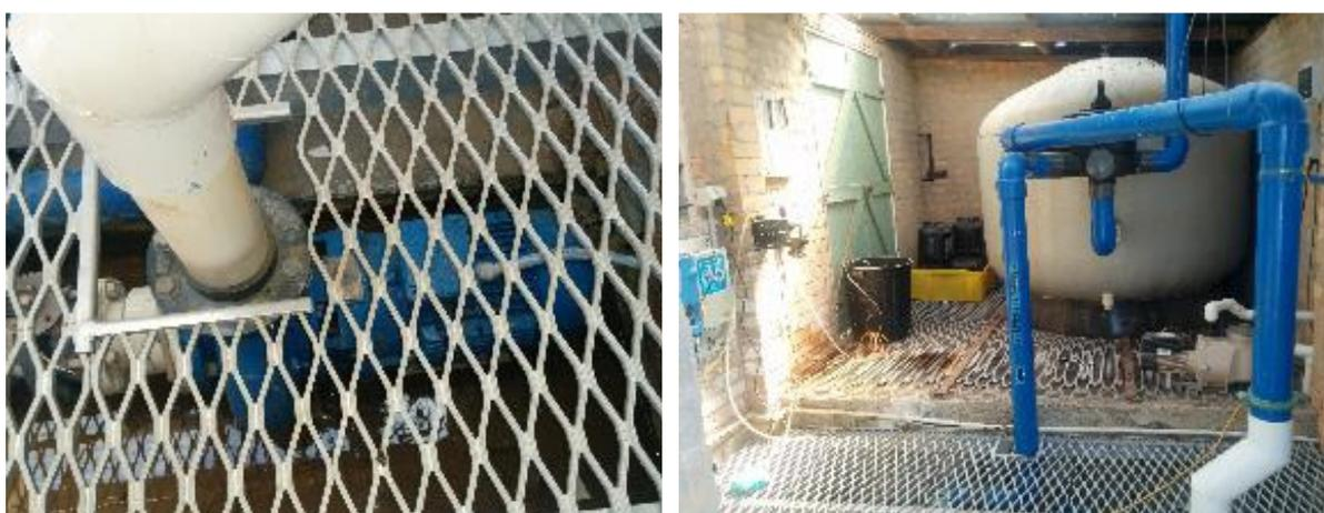
**Reticulation pump & motor set under grate with filter cell in plant room**
