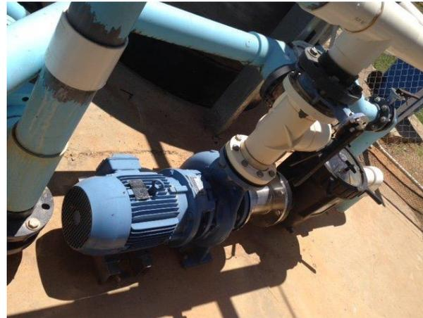
**Reticulation pump/motor set & strainer open air.**
