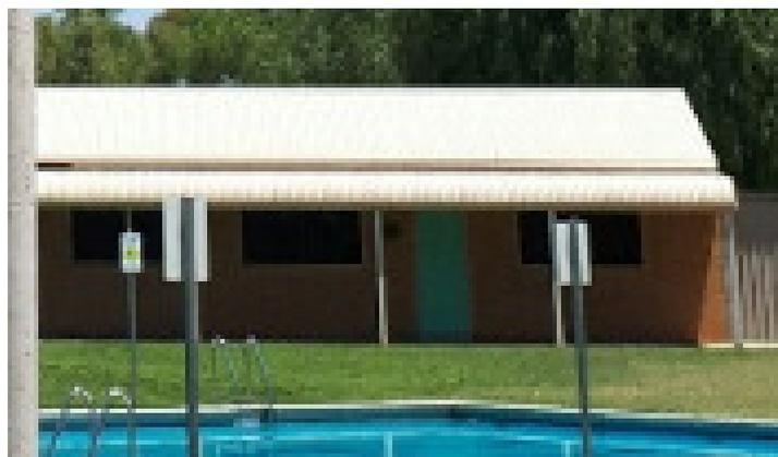
The Swimming Clubrooms are constructed of brick with an iron roof and veranda. The building is in very good condition but does not provide DDA access.
