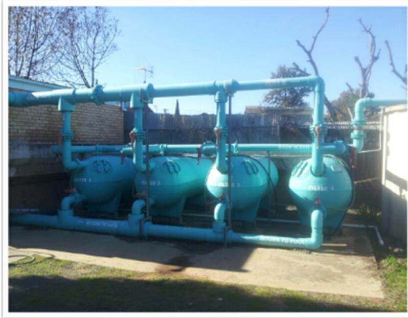
**High volume horizontal sand filters with associated pipework**
