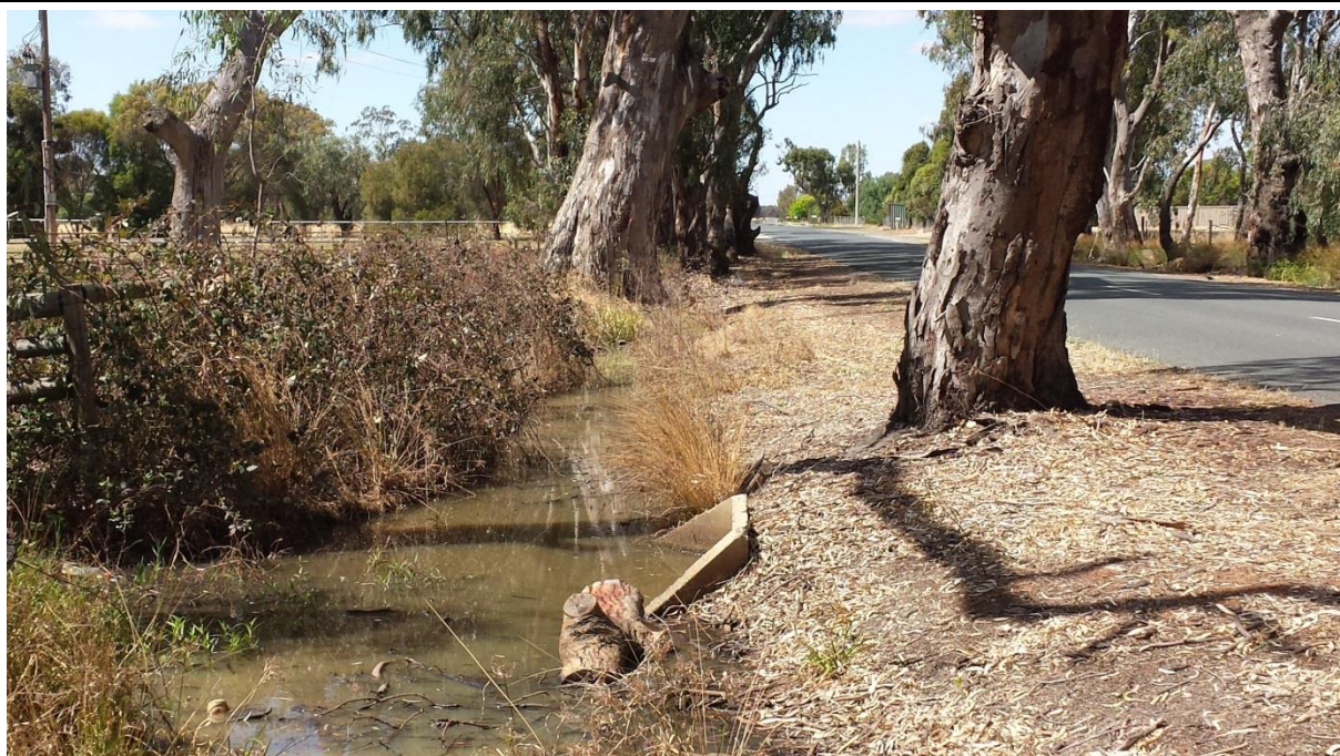
Photo 1 – Mary Ann Road (North of Brecon Court) showing water held adjacent to culvert at floodway
