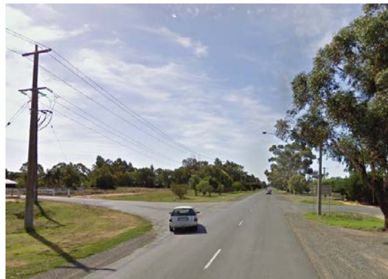
Figure 2.2: Difficult to Cross – McEwen Road (Google)
