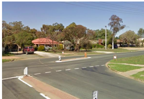
Figure 2.4: Absence of Connecting Facilities – Bowen Street (Google)
