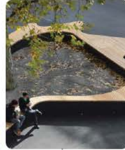
DDA TIMBER SEATING ON CONCRETE EDGE
