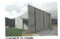
CONCRETE TILT PANEL
