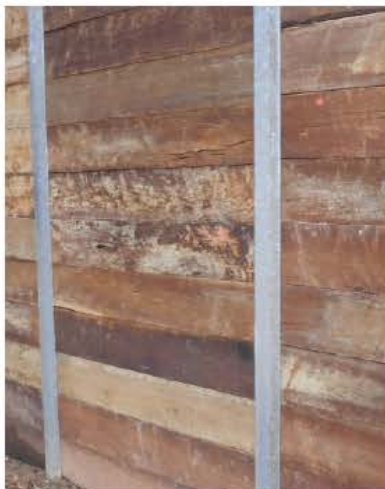
RECYCLED TIMBER AND GALVANISED STEEL
