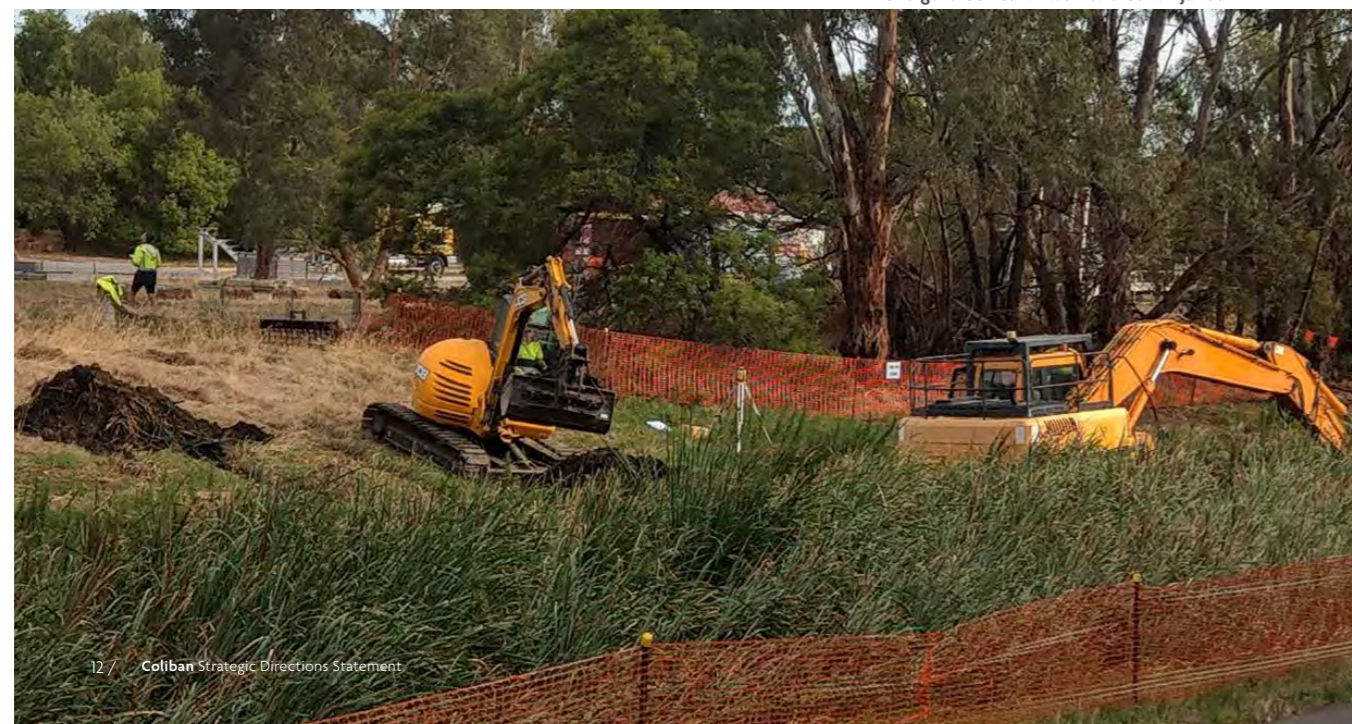
Bendigo Creek earth works. Credit: Djandak
