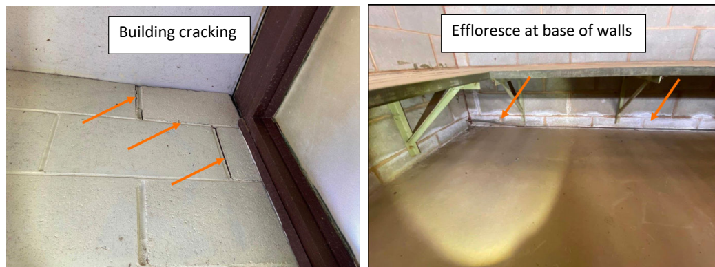
Figure 5 Rochester Pool Condition (Source: FMG Engineering, 2022)
