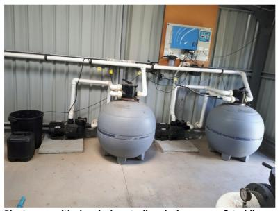
Plant room with chemical controller, dosing pumps & toddlers pool filters.
