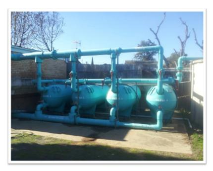
High volume horizontal sand filters with associated pipework
