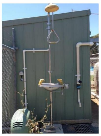
Sodium Hypochlorite Shed with eye wash attached
