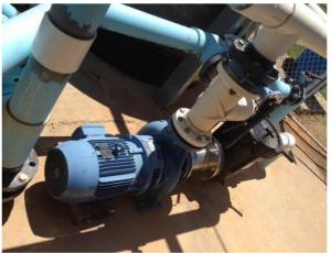
Reticulation pump/motor set & strainer open air.
