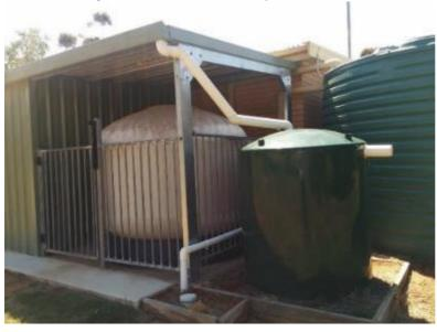
Filter & weather protection structure with small rainwater tank (front) & backwash tank
