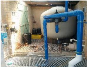
Reticulation pump & motor set under grate with filter cell in plant room
