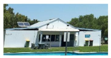
The amenities are constructed of brick with the kiosk in the middle and the amenities each side. They are in an average condition and will require a major upgrade to be DDA compliant. The kiosk requires a full internal refit.
