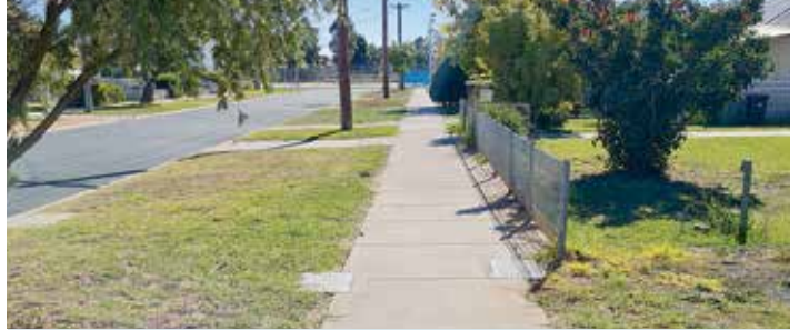
A section of footpath in Cox Avenue, Tongala has been replaced.
