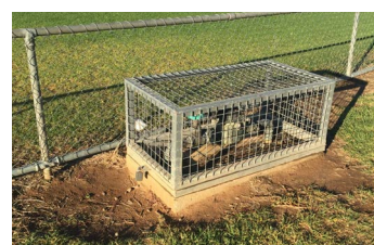
Water meter cage example
