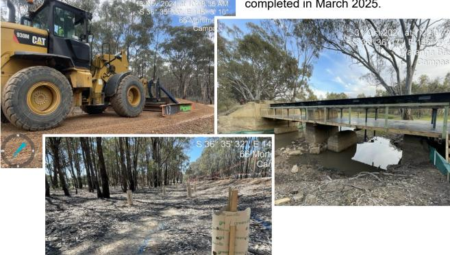
Construction of the asphalt path in Rushworth will re-commence at the end of November. Pausing the works for several months has given the sub-base sufficient time to dry and strengthen. It recently passed the required proof roll test so the base layer and asphalt can now be installed. These works are scheduled to be completed in December 2024
