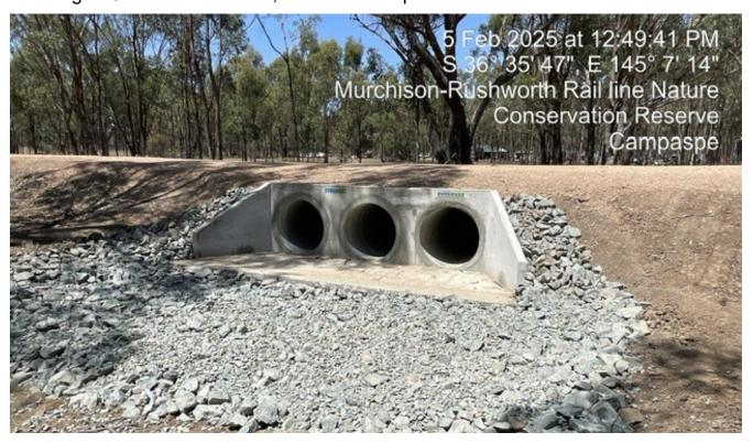
Repairs to a large three cell culvert was completed in January (image above), and repairs to six VicTrack bridges are also underway. Three of the bridges require new concrete decks. These are being manufactured throughout February and are expected to be installed in mid March. The contractor, Northern Constructions Group, are also installing safety balustrading, regulatory signage, fencing and bollards.
